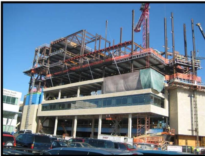
deck. The foundation is a mat padding. On top of the roof, there is a large penthouse which holds the mechanical equipment which is all supported by the steel framing of the building. For lateral loads, cross bracing is integrated within the frame.
